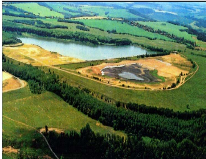
Remediation site Seelingstädt
