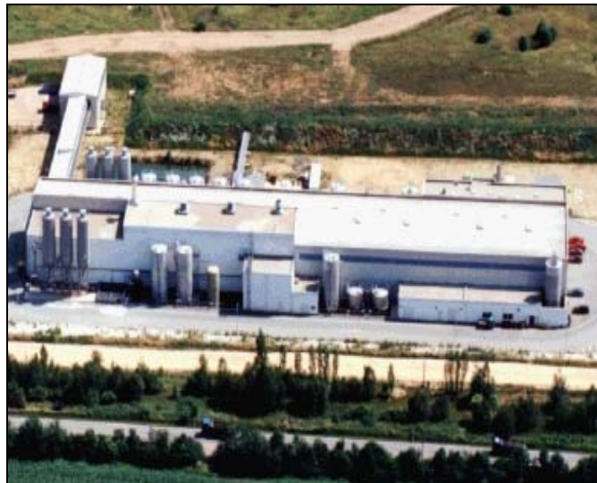
Air view on new built water treatment plant Helmsdorf
