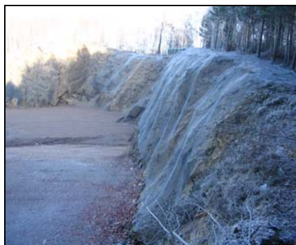
temporary facerock protection
