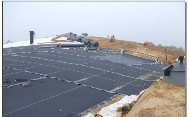
Geomembrane and drainage mat sections 2/3
