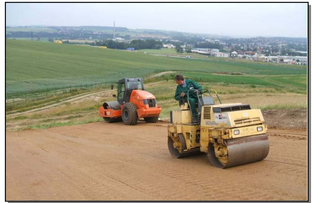
Installation of mineral sealing layer cell 1
