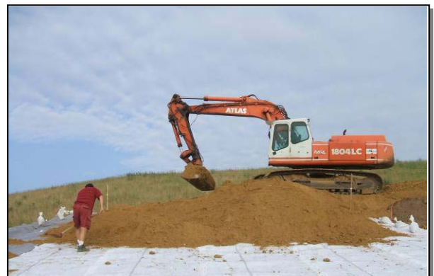
Placement of reclamation soil section 1
