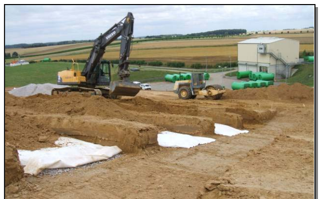
Trenching for the passive landfill degasification
