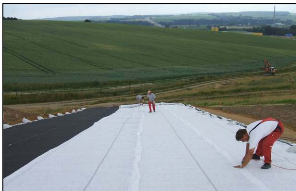
Installation of geomembrane and drainage mat cell 1
