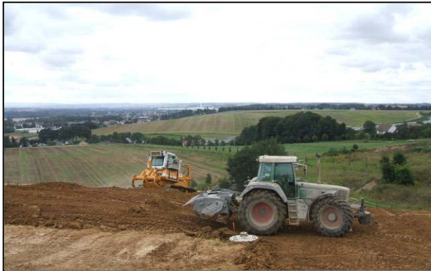
Strengthening of applied mineral sealing layer sections 2/3
