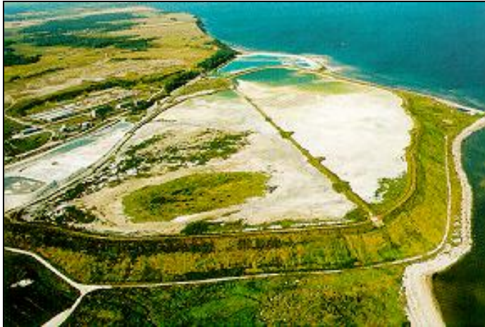
Sillamäe Radioactive Tailing Pond in 2000
