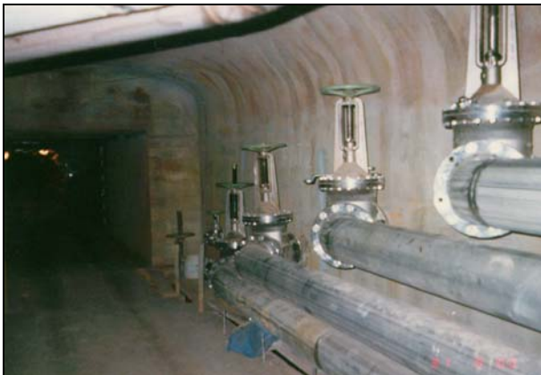
Pipelines are crossing the concrete plug body
