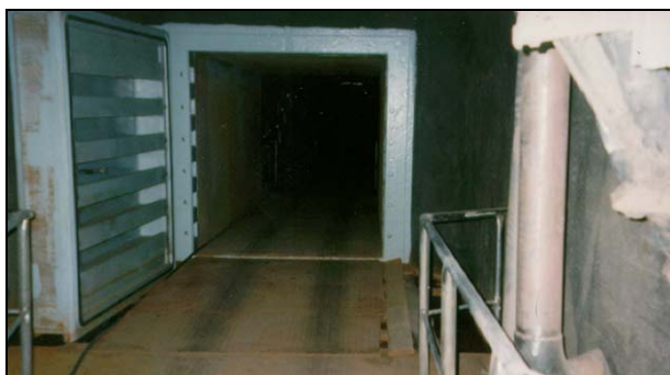
Concrete plug with dam door for backwater pressure of 23 bar
