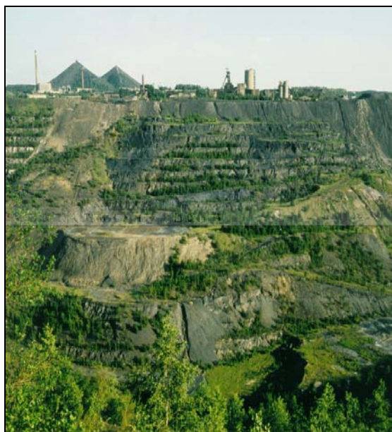
Former uranium open pit mine Lichtenberg
