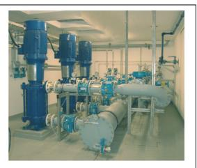
Removal of the existing aggregates and pipework to elevated tanks of Elbingerode, construction of piping and pump systems including clean water pump station.
